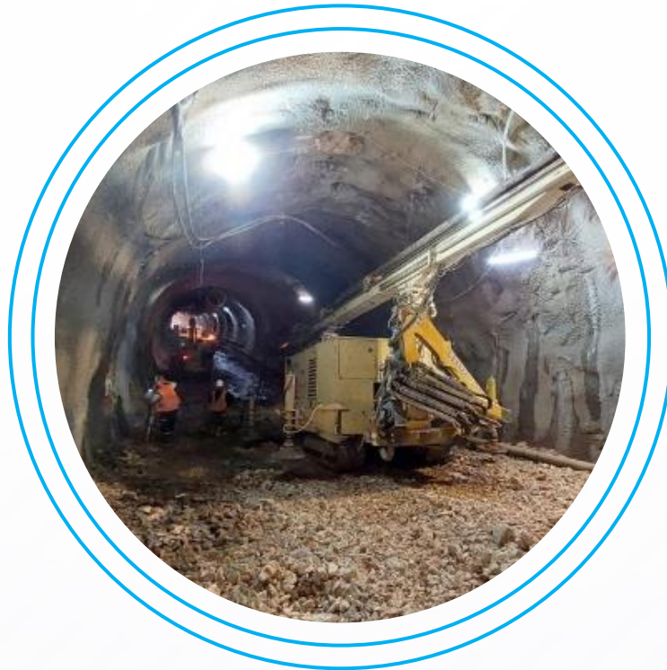
The main entrance tunnel
