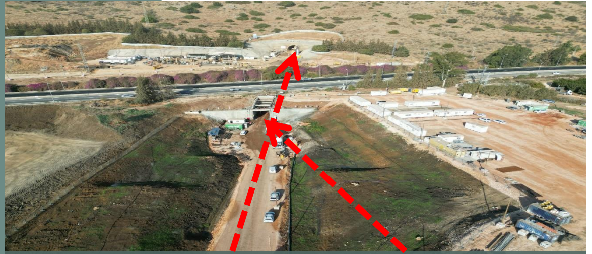
View of the MAIN ENTRANCE PORTAL and LOW PRESSURE PORTAL
